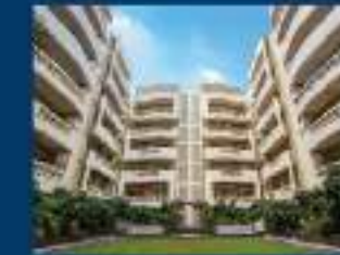
SHALIMAR DWELLING AP SEN ROAD LUCKNOW
