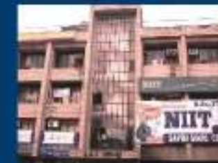
SAS HOUSE SARPU MARG LUCKNOW
