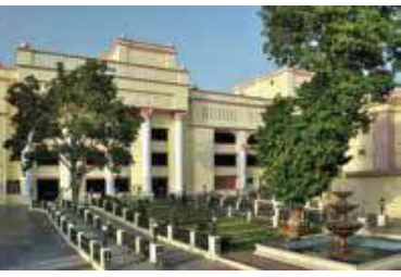
MULTILEVEL PARKING, HAZRATGANJ, LUCKNOW
