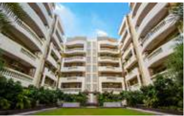
SHALIMAR DWELLING, AP SEN ROAD, LUCKNOW
