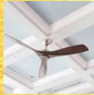
CEILING OIL BOUND DISTEMPER
