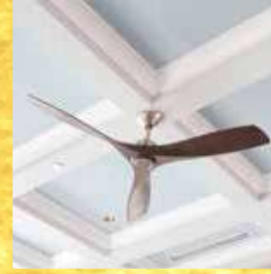
CEILING OIL BOUND DISTEMPER
