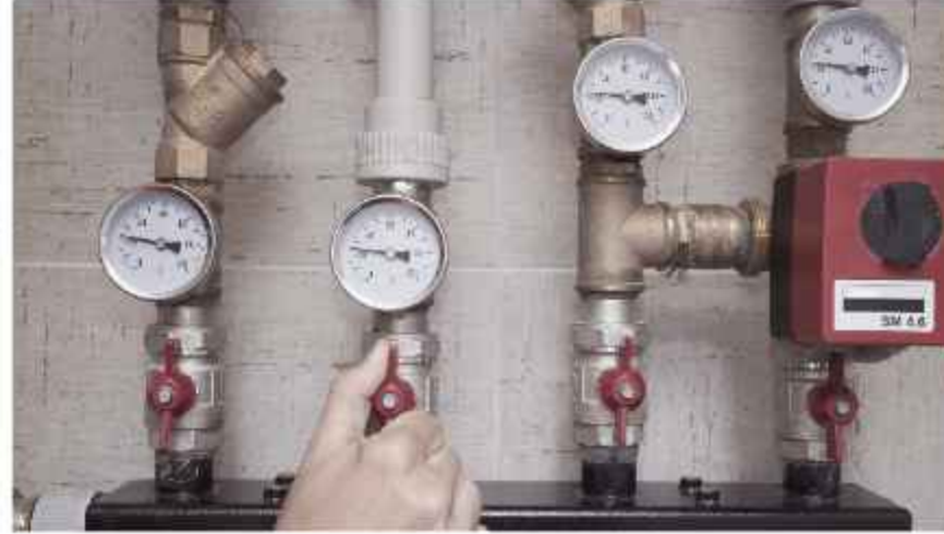
Smart Metering for Water and Electricity
