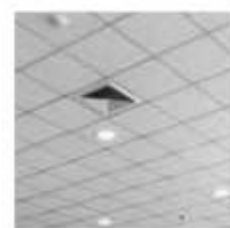
CEILING GRID FALSE CEILING
