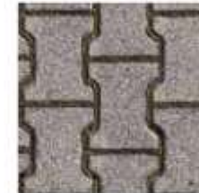
INTERNAL ROADS INTERLOCKING BLOCKS/ TREMIX CONCRETE ROAD
