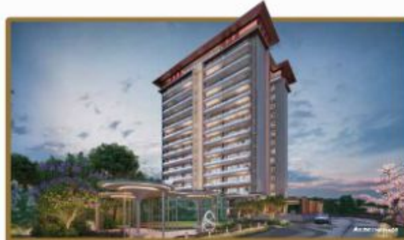
Eldeco Skywalk, at Eldeco City, IIM Road, Lucknow
