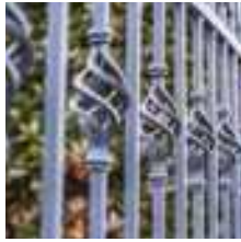
RAILING MS RAILING WITH ENAMEL PAINT FINISH
