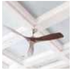
CEILING OIL BOUND DISTEMPER
