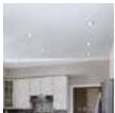
WALL / CEILING OIL BOUND DISTEMPER
