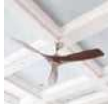
CEILING OIL BOUND DISTEMPER
